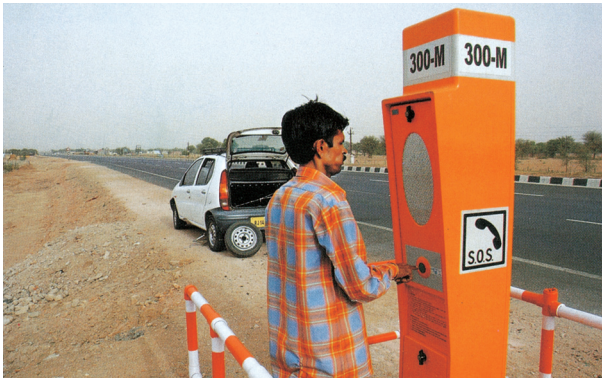
Fig. 7.10 : Emergency call box on NH-8
