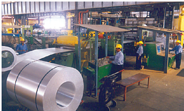
Fig. 6.3: Strip coating mill at smelter of NALCO
