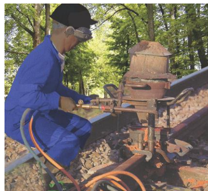
Figure 3.11 Thermite process for joining railway tracks
